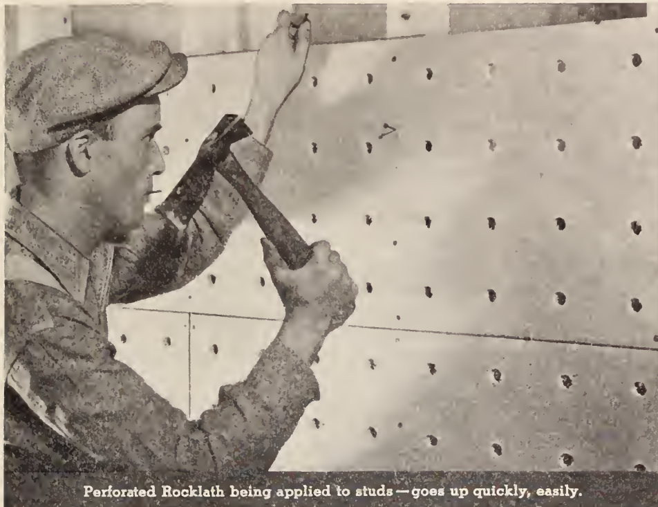
Plaster penetrates holes — gets strong, extra grip on back of lath.
